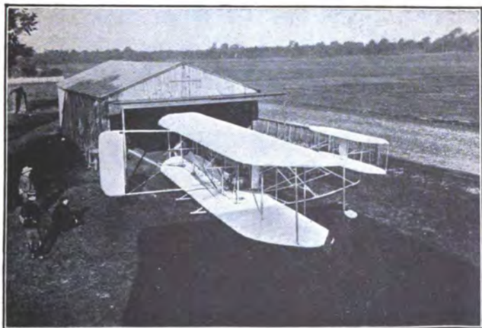
WILBUR WRIGHT'S AÉROPLANE outside the hangar at Le Mans, showing main supporting surfaces horizontal rudder at right, vertical rudder at left.
