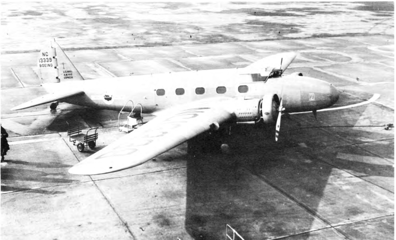
Wearing the livery of United Air Lines, c/n 1721 is seen at Boeing Field in 1935 before being modified to 247-D standard. Note the 2-blade controllable pitch propellers and Air Express insignia on the nose. (G. S. Williams)
