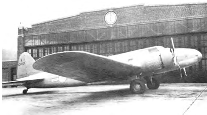
The second of three tail configurations tried on 1682 in 1934 and modified engine nacelles. (G. S. Williams)
