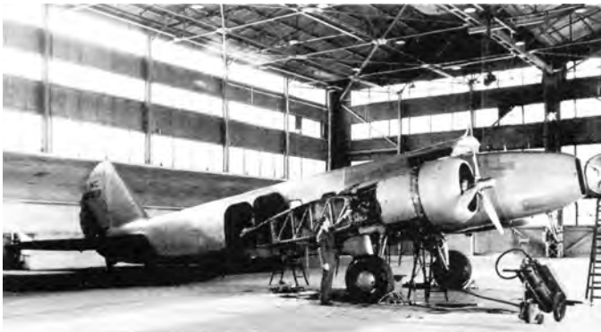
About 1946, c/n 1694 had extra fuel tanks installed and other rework done at Boeing. (Photo - Boeing #H5160)
