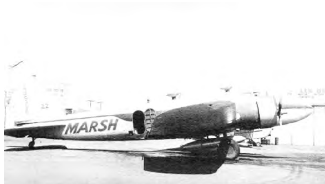
C/n 1729 with modified nose, extra radio equipment and spray attachments. (Photo - Peter M. Bowers)
