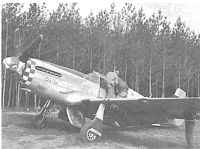
"Sally", also 505th Fighter Squadron, bears damage to her nose and left wing from snuggling up too close to a balloon cable. Serial number 42-106579.
