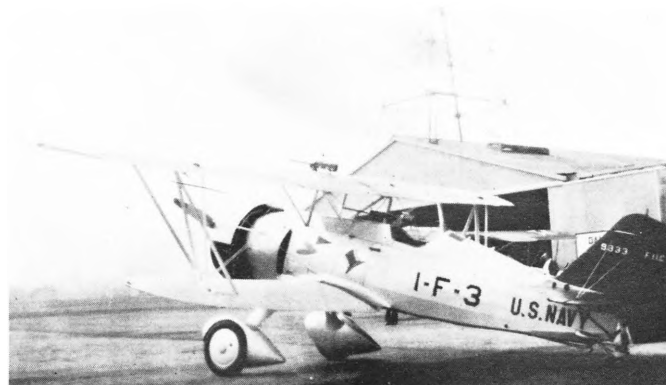
A second 1-F-3, 9333, at Long Beach on 18 February 1933. Note lower half of cowl painted red and 16mm camera gun mounted on top of the wing. (Photo - Ed McCollon)
