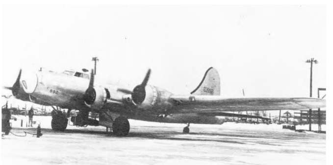
83992 was listed XPB-1 when used by Cornell Aeronautical Laboratory as a test vehicle. Note Westinghouse J-30 jet engine below bomb bay. (Photo - Cornell AL)
