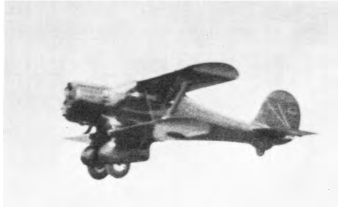
Not positively identified as C/N 1 or 2 but probably the latter with fixed tailwheel. This was not revised on C/N 2 as Pilot Ross became used to handling the airplane with the fixed rear wheel. (Photo - Bowers)
