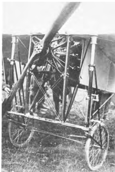
An example of the very small diameter twin-row Gnome Rotary Engine installation in a Bleriot XI.
