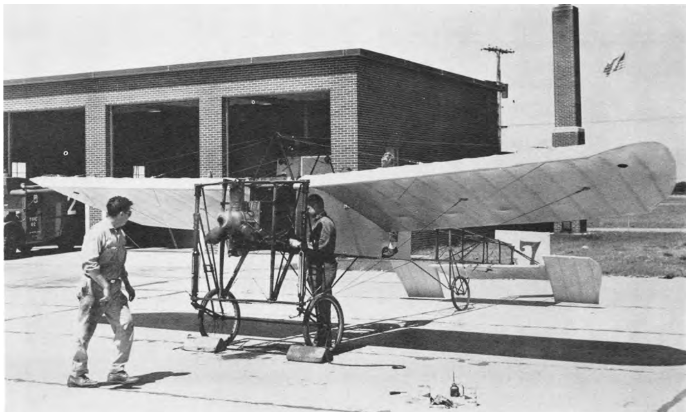
The Palen Bleriot XI being tuned. Note that the engine is forward of the "bedstead".
