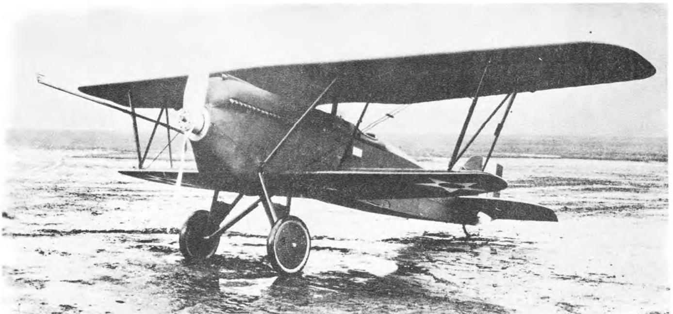
The first production PW-9D airplane, No. A.S. 25-295 with long airspeed boom for test. (Photo - USAF 8450 AS)
