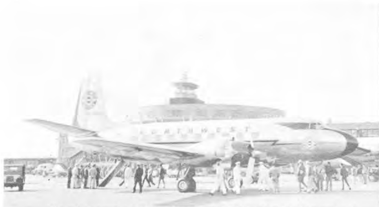
The first of the Northwest Airlines Martinliners. It shows the original wing configuration, (3° dihedral) and small vertical fin. (Photo - Dave Gauthier)
