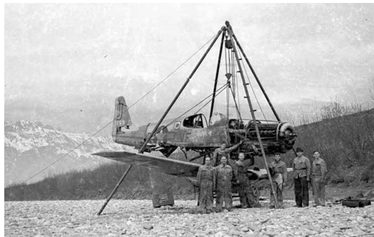
A salvage crew hoisting 43-24853 to remove the wings and place the components on carts for removal from the river bed.
