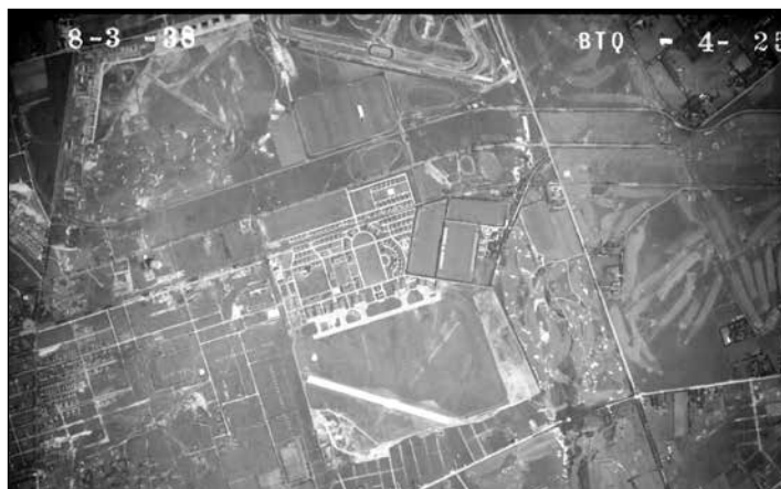
By August 3, 1938, the construction of the first paved runway at Mitchel Field is almost complete. (USAAC photo)
