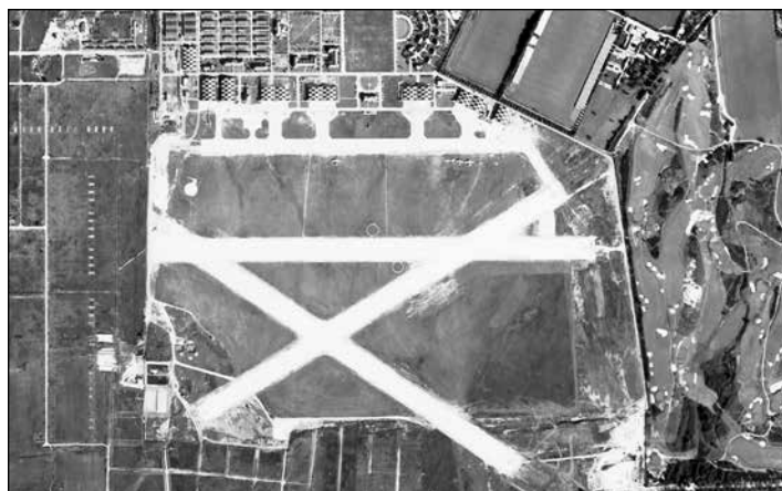
And by September 1940, the third paved runway was complete. (USAAC photo)
