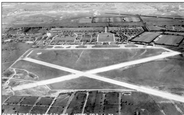
By July 1939, the second paved runway had been completed. (USAAC photo)
