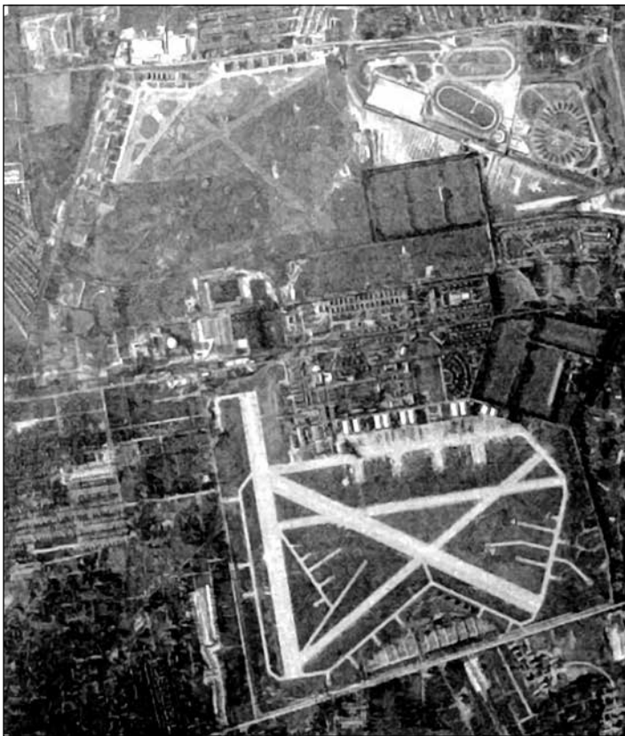
During WWII, a fourth paved runway was added along with hard stands for aircraft dispersal. This 1948 photo shows Mitchell Field in pretty much its final configuration. (USAF photo)
