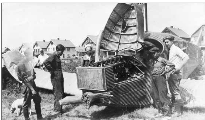
The first JL-6 "built" (assembled) by J.L. Aircraft was test flown on March 24, 1920, by Emil Monz at Roosevelt Field, Long Island, New York. It was damaged beyond repair following an engine failure. (AAHS archives, Gerald Balzer collection)
