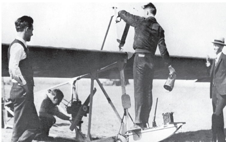
A CG-2 fitted with a 10-hp Cleone engine.
