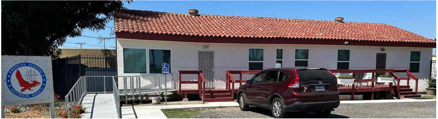
ABOVE: The refurbished AAHS offices sporting a new coat of stucco and new windows.
