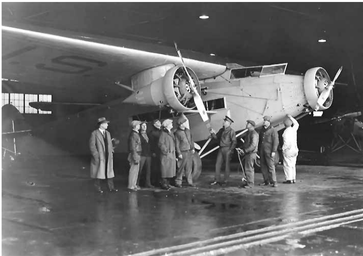
The 28-126 as modified on Wright Field to take the new Wright R-975 engines and redesigned as XC-7 with tail number XP545.
