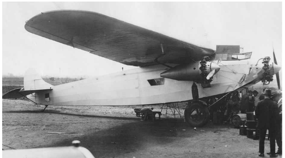
The completed Trimotor for Byrd, still unpainted and before its first flight in May 1927.
