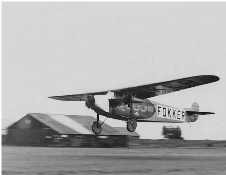
The first F.VII/3m during a test flight over Schiphol Airport. Note the original large tail fin.
