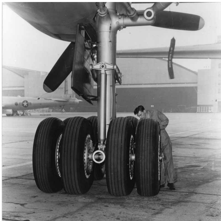
Multiple-wheel bogie landing gears were commonly used later to increase the landing footprint of large aircraft, but they were first used on B-36s, as depicted here on B-36A 44-92015, and the XC-99. (AAHS-d022397 from the NARA collection)
