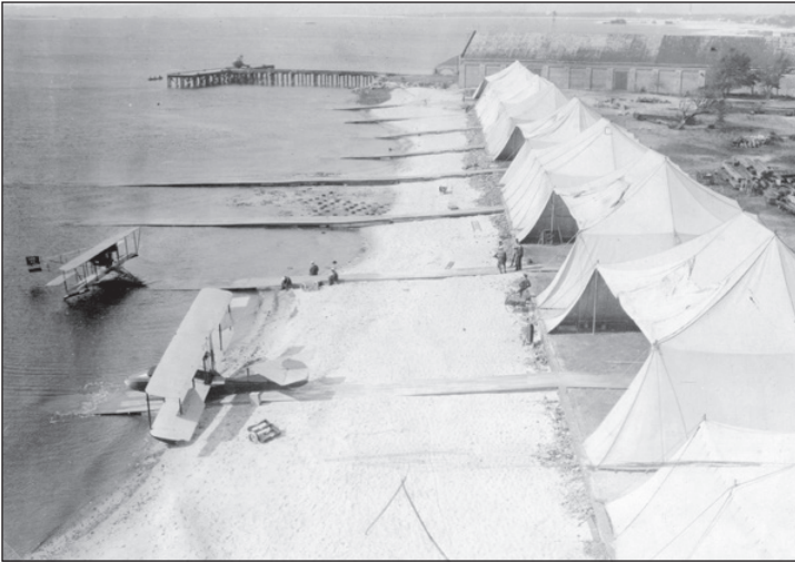
The birth of naval aviation at Pensacola started with the establishment of a seaplane base with tent hangars in 1914. (Naval History and Heritage Command)
