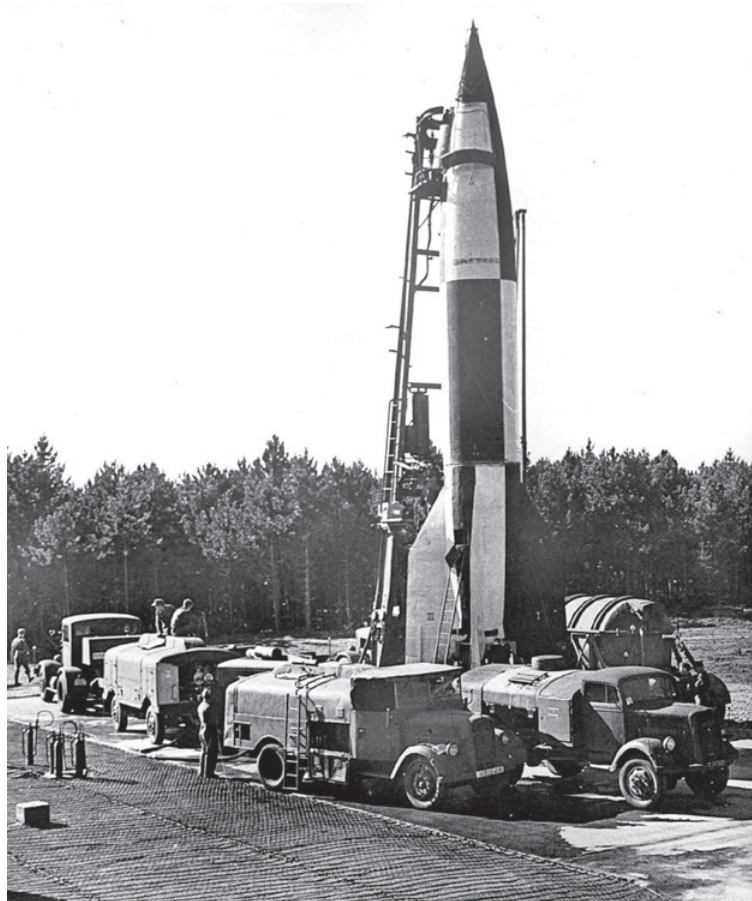
A Photo illustrating most of the support system required to transport, prepare and launch a V-2. (IVM/U.S. Army Archives via Rare Historic Photos)
