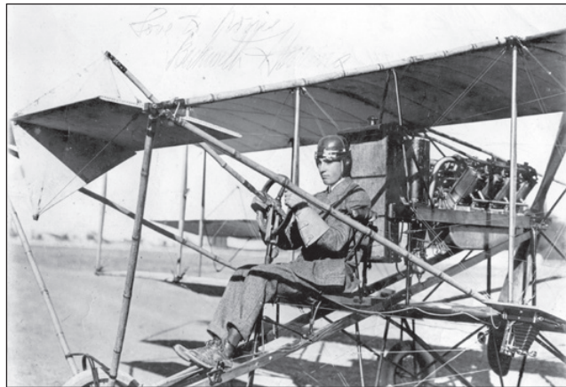
At the Texas State Fair in Dallas, Tex., in 1911, Havens' became one of the earliest known aerial photographers when, with the help of a local news photographer a Kodak camera was mounted (lower right portions of the photo) on the leading edge, allowing Havens to snap one photo on each flight he made around the area. (Photo from Wikipedia commons)
