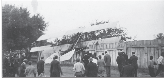
Minor mishaps were closer to the rule than the exception, with crashes due to various causes also taking a toll on machines and aviators. Here it appears that the aircraft didn't achieve sufficient speed to clear the fence and tree and settled back on its tail on the fence. (Photo from San Diego Air and Space Museum)
