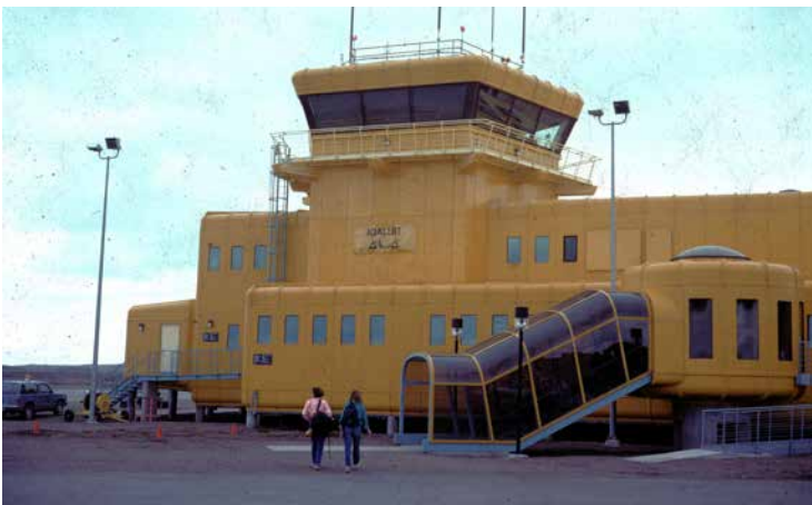
Control tower and related aviation facilities, Frobisher, 1989. Frobisher is the largest settlement in Canada’s eastern Arctic.
