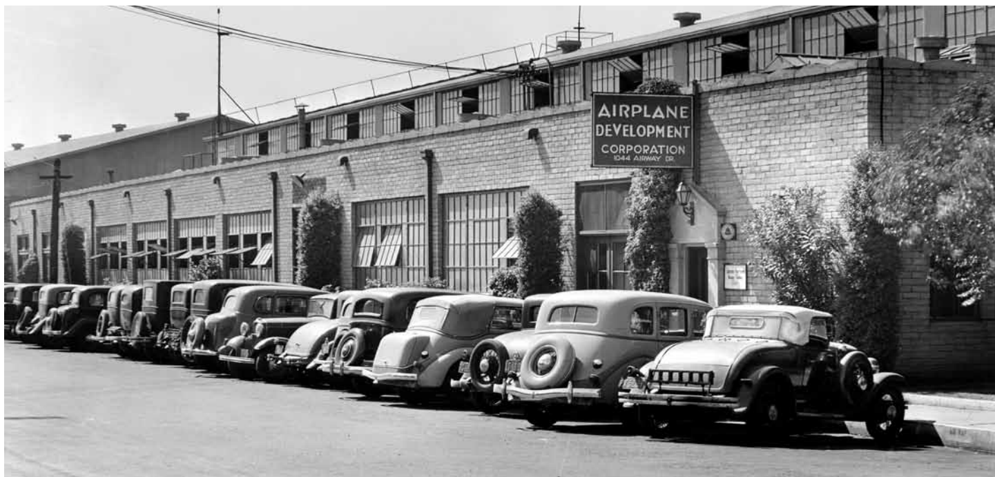
Cars parked in front of the administration and design office buildings of the Airplane Development Corp. (ADC) factory. (Photo from the Gerald Balzer collection, AAHS)
