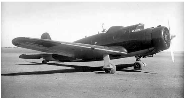
One of three V-1As transformed into bombers by the Spanish Republicans at the Leon base. These planes were armed with three machine guns and bomb launchers under the wings. (Photo from the Juan Arraez Cerda collection)
