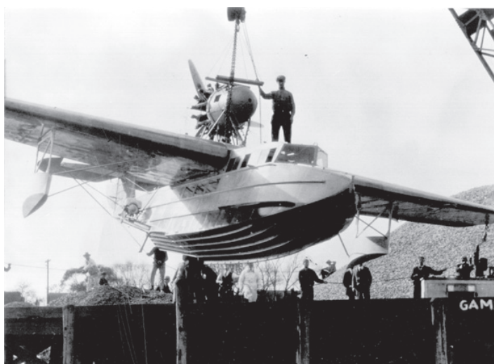
The prototype of the F-11 with its early type small floats is hoisted into the water. An outboard motor facilitated taxiing. (American Fokker photo from the author's collection)
