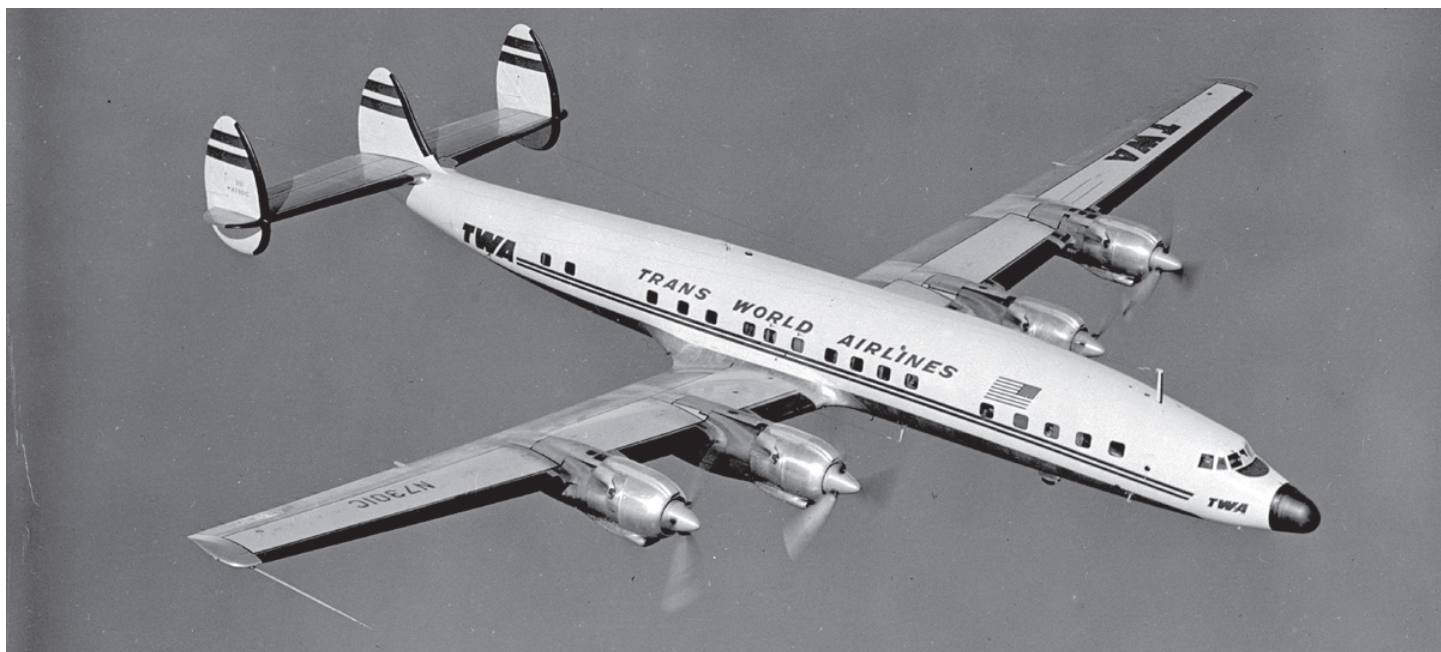
View showing TWA Lockheed 1649A's high-aspect ratio wing. (AAHS photo archives, Eric Miller collection, AAHS-1633)
