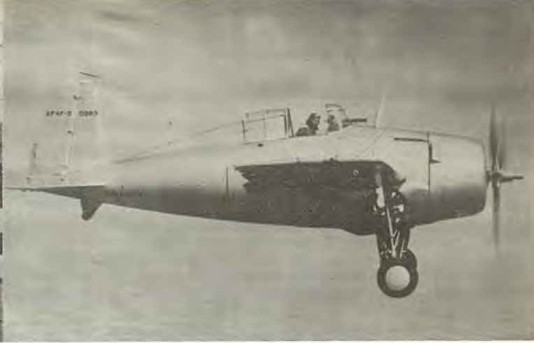
F4F-3 in landing condition. Landing gear design was a carryover from F3F. Photo - Navy No. AN-53021, 4-3-39.
