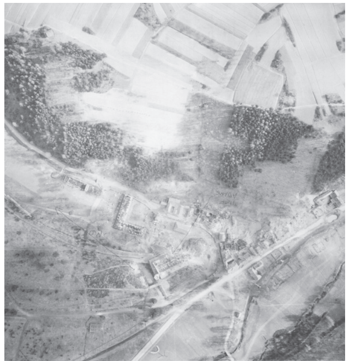
This is a bomb assessment photo taken shortly after the raid showing the destruction of the complex. Difficult to make out is a penciled track from the upper right to lower left across the center of the complex labeled "Dief / Adams." (USAF photo from the A.J. Diefendorf archive)
