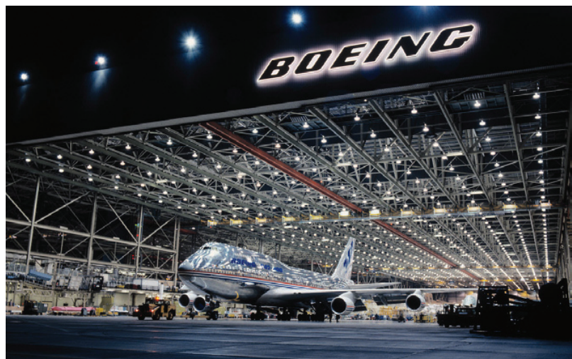
Boeing was not only creating a brand new aircraft design, they also had to build a completely new facility in which to build it. The Everett, Wash., factory where the 747 is built is still the biggest building in the world by volume. (Photo from the Boeing Company)
