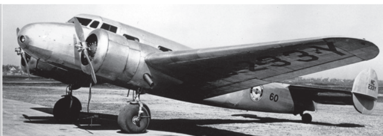
First Lockheed Electra after original forward sloping windshield was replaced. (Lockheed photo from the author's collection)
