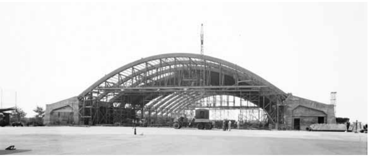
The 1943 Republic Aviation final assembly hangar nearing completion. This building is now Hangar 4 at Republic Airport housing Invictus Jets. (Courtesy of Republic Aviation Archives via LIRAHS)
