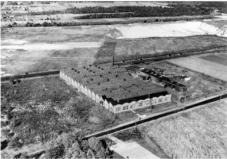
This aerial view shows the former Fulton Truck Factory in 1927, which was used by McAvoy Homes inc. just before Sherman Fairchild bought the property and developed his factories and flying field there. The factory lies between the Long Island Railroad (LIRR) and Conklin Street. Sherman Fairchild built pontoons in this building in 1927. (Courtesy of the Long Island Republic Airport Historical Society (LIRAHS))
