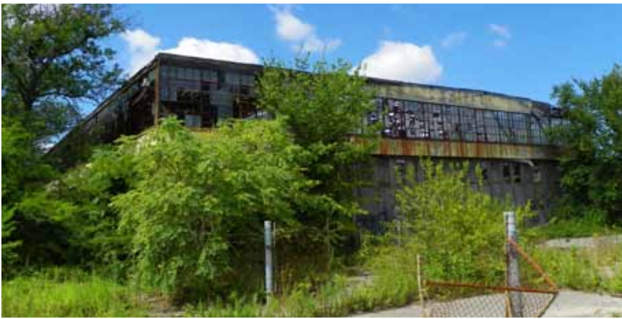
Building 5, the original 1928 Fairchild Airplane Manufacturing factory, in one of the last remaining historic Fairchild Republic Co. building still intact, although gutted. It has been abandoned since 1987. (Courtesy Ken Neubeck)
