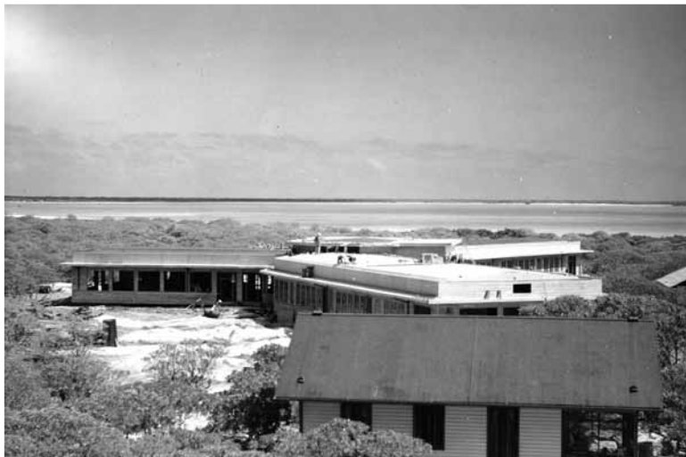
Pan American Airways, Wake Island accommodations under construction. (Photo from the editor's collection)
