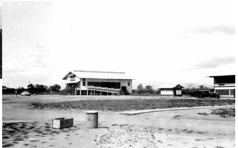
One of the most frequented facilities on the station, the Base Theater, also doubled as a classroom for the Training Center and permanently assigned units. The concrete walkways were a Godsend. (Richard W. Spencer)
