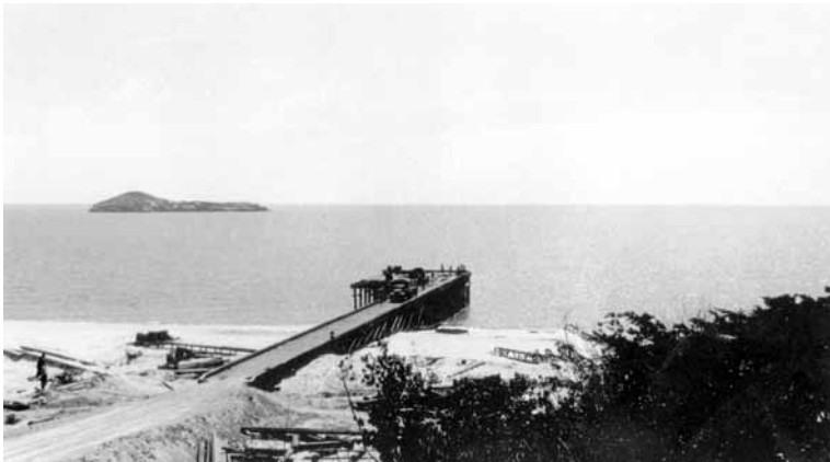
The pier constructed with some difficulty by the 11th Engineers looking south near the end of the Rio Hato Air Base primary. The beach dropped off to great depth very quickly near Rio Hato. Once constructed, it was actually rarely used – except for swimming, diving and fishing. The small island in the distance had a Spanish name, but was universally known, well into the 1960s, as "Bird Shit Island," and when the prevailing winds were just right, the smell was truly amazing! It was the object of frequent Coast Artillery and Aerial Bombardment training, much to the enjoyment of personnel garrisoned there. (Richard W. Spencer)
