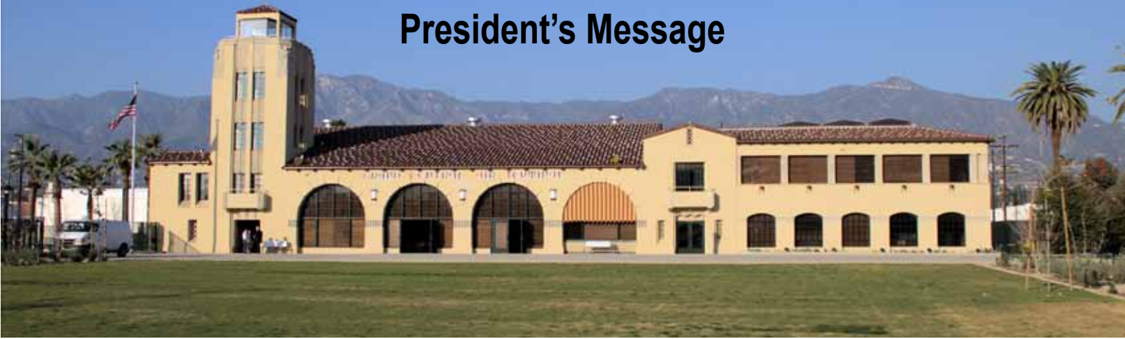
Restored Grand Central Air Terminal west side. (Photo by Hayden Hamilton)
