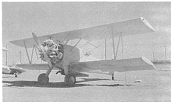
Ross Dusters use Stearman PT-17s and NAF N3Ns that have been modified with an R-985 engine.
