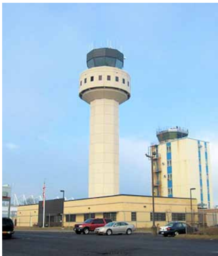
The FAA replaced the existing 1962 control tower in 2003 with the 157-foot cylindrical tower.
