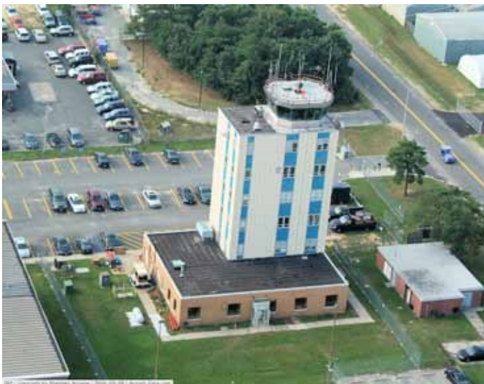
In 1963, the FAA built this seven floor tower, which also housed the New York Air Route Traffic Control Center.
