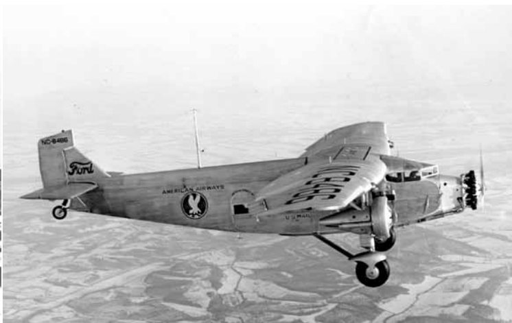
Ford 5-AT-C, NC8486, in typical American Airways markings. This particular ship was a bit unusual, having been built as model 6-AT-A and used by Ford Motor Co. for about a year before American bought it. (Photo courtesy American Airlines Museum)
