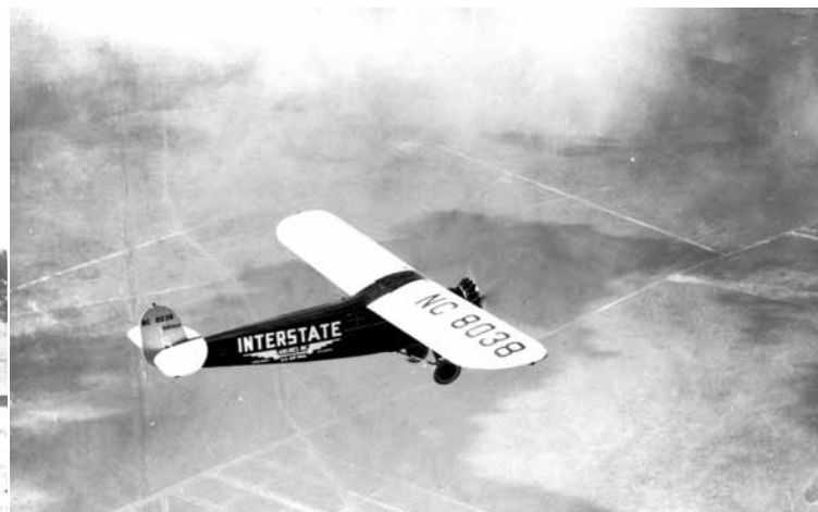
Fairchild FC-2W2 NC8038 in flight along CAM-30. This Wasp-powered version of the Fairchild cabin monoplane carried mail and/or as many as six passengers. (Photo courtesy Fairchild Republic Co.)
