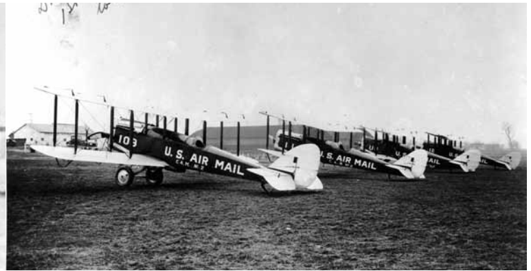
Robertson Aircraft Corp. began CAM-2 airmail service with these revamped WWI DH-4s. The smartly-painted ships (maroon fuselages, silver wings and tails) began round-trip operations on April 15, 1926.
