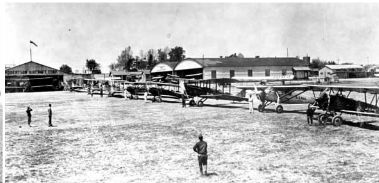
Robertson Aircraft Corp. aircraft and facilities at Lambert Field, ca. early 1928. The three aircraft at right were all used on CAM-2 airmail service. From right: Travel Air 4000, Ryan Brougham and de Havilland DH-4. Note the profusion of other aircraft (Wacos, Standards, DH-4s, etc.) used by the Robertson organization for flight training, aerial photography, charter, and so on. (Photo courtesy Betty Robertson Uhl)
