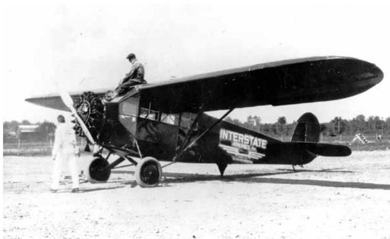
Fairchild FC-2 NC6692 was Interstate Airlines' first aircraft. Ship was powered by a J5 Whirlwind and could carry four passengers. (Photo courtesy Fairchild Republic Co.)
