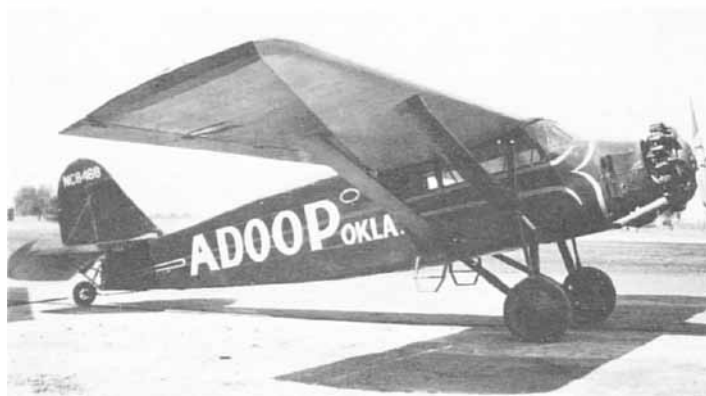
SM-1F DETROITER (6PCLM, 300-hp Wright R975A). 1929 production; last SM-1 variant. Built under ATC 136.
