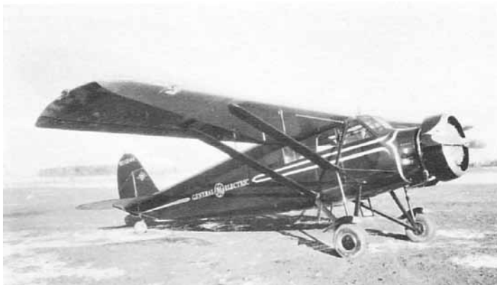
MODEL "W" JUNIOR (Same as SM-7 A with minor changes). 1932 production; 5 built under ATC 435: s/n 3050 thru 3054.
