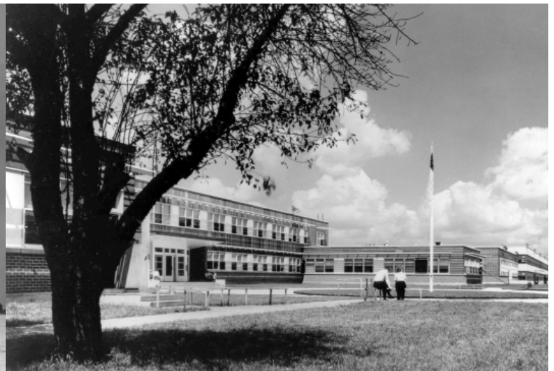
The administration building. The original building was completely destroyed by fire on July 18, 1944, but had been completely rebuilt by the following October. (Photo from the Des Plaines Public Library collection)
