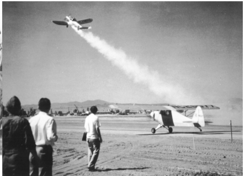
JATO charges bolt the Ercoupe off the March Field runway in August 1941, an early step in the American military's development of rocketry that gained momentum in the latter stages of WWII. (NASA photo)
