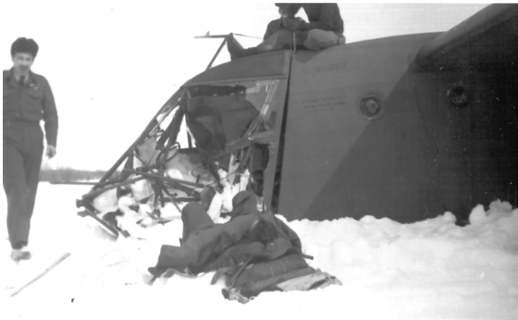
Waco CG-4A USAAF glider number one, crash landed on a small lake near the Petitot River. Injured pilot lies on cushioned ground with severe back injuries. The cargo is an M-29 Weasel that appears to have shifted forward during the hard contact with the lake ice. Men atop the wrecked forward fuselage are prying the upper hinge loose to remove the nose unit and extract the Weasel. (Photo: AINA Image 20080-4)
