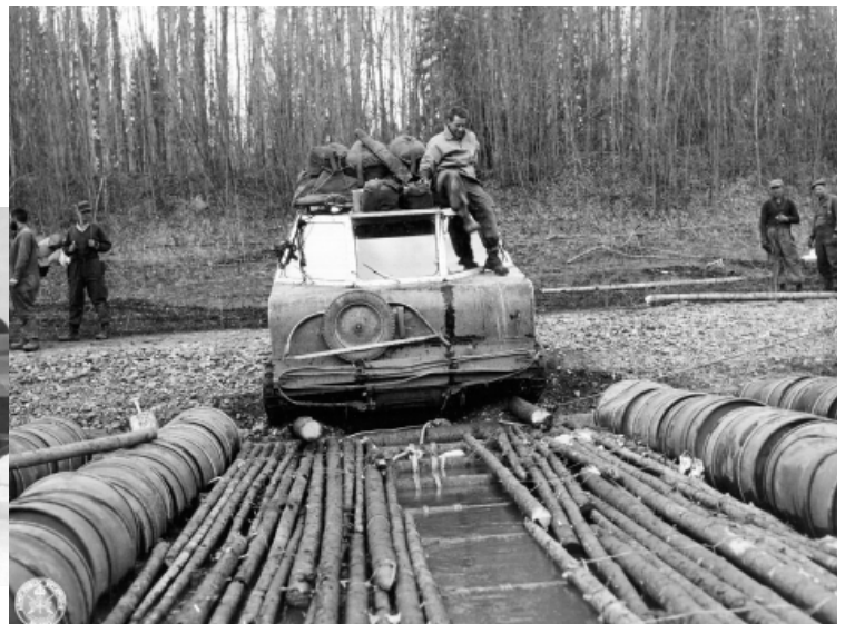
Engineers have constructed a log raft for snow machines to cross the Fort Nelson River. The vehicle's roof is loaded with necessary equipment lashed down to prevent shifting while traversing rough terrain. (Photo: AINA Image 20104)
