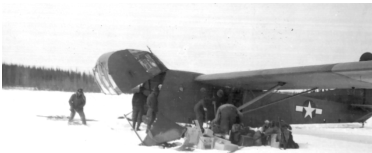
Waco CG-4A USAAF glider number one, crash landed on a small lake near the Petitot River. Injured pilot lies on cushioned ground with severe back injuries. The cargo is an M-29 Weasel that appears to have shifted forward during the hard contact with the lake ice. Men atop the wrecked forward fuselage are prying the upper hinge loose to remove the nose unit and extract the Weasel. (Photo: AINA Image 20080-4)
