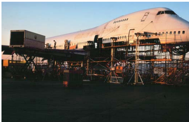
Huge jacks and cross-beams are all that support the front of JAL8122 as skin, stringers, formers and forgings are removed and replaced. The AOG Team was divided into two 12-hour shifts and worked hard to beat the rapidly approaching cold autumn nights so common to Alaska. (Photo by the author)
