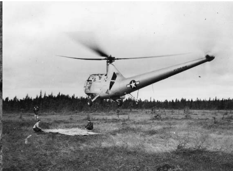
HOS-1 landing at the lakeside platform bringing one more survivor of the SABENA crash to be ferried by life raft to a waiting PBY floating on the lake. Platforms were necessary to prevent helicopter's landing gear from sinking into the muskeg. (Photo from the author's collection)
