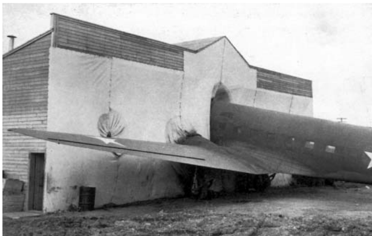
A representative photo displays a more permanent nose-hangar with canvas front cover having four engine cutouts capable of handling a C-54. (USAAF photo from the author's collection)
