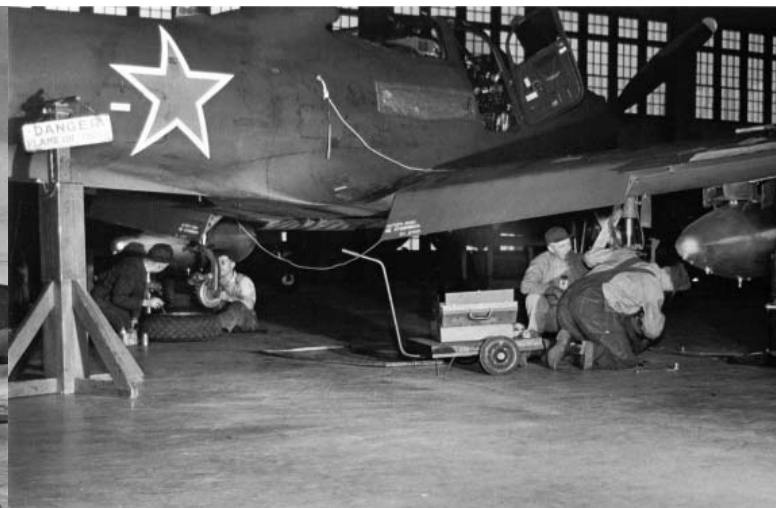
Soon after the Alaska-Siberia Route began the CWTD unit was reportedly evicted from Hangar #1 enabling lend-lease P-39s and P-63s to be maintained prior to the stubborn Russians accepting aircraft with all "squawks" cleared of the logbooks. Mechanics are working on a P-63's wheels or brakes. (Photo from the author's collection)
