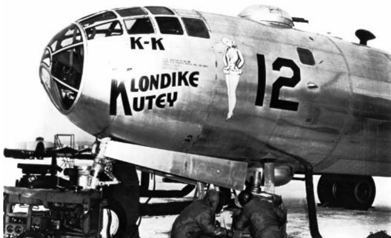
Maintenance crews with help from a Jeep Heater appear to be working on Klondike Kutey's nose landing gear. (USAAF photo from the author's collection)
