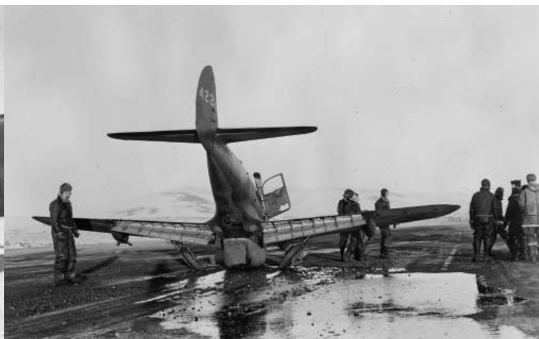
Bell P-39 suffers a nose-gear collapse at Nome, Alaska, the last fuel, maintenance stop before flying across the Bering Sea to Eastern Siberia. (USAAF photo from the author's collection)
