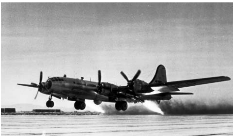
This B-29 was modified to use multiple racks of JATO units for "hot n' high" or short runway operations at maximum gross weights. Other B-29s were subjected to numerous modifications such as several different aerial tanker configurations among other classified missions worldwide both during late WWII and the postwar years. (USAAF photo from the author's collection)
