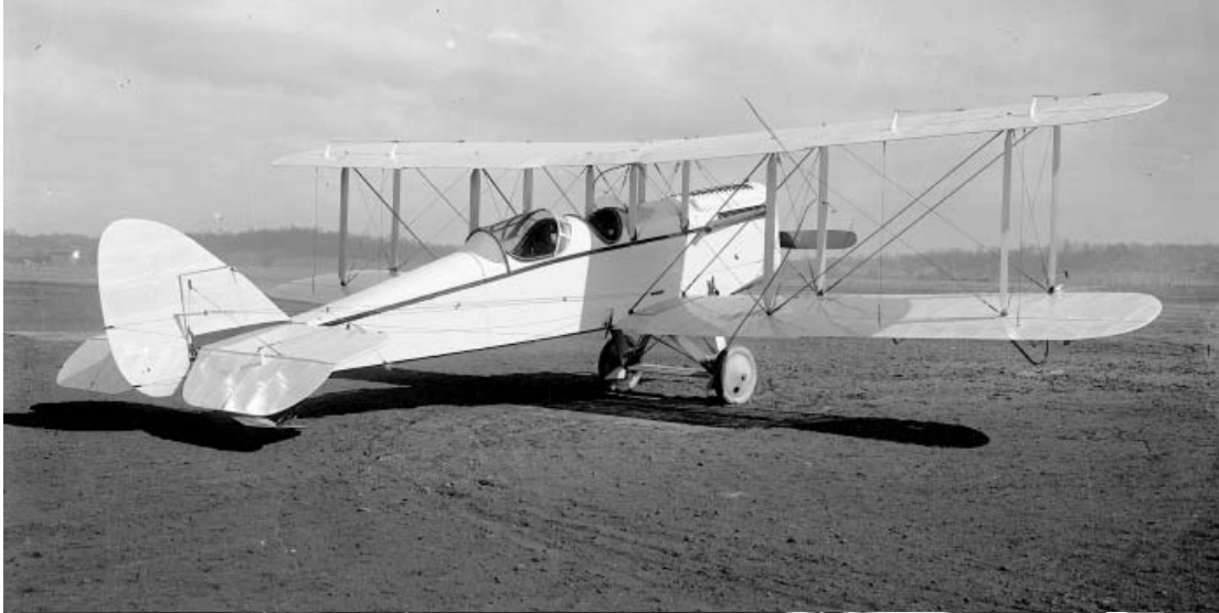
Dayton-Wright modified at least one DH-4 into a three place ship - two passengers, one pilot. The passengers rode in a cozy enclosed cabin and the plane became known as "The Honeymoon Express" as a result. (Photocourtesy of Special Collections and Archives, Wright State University, MS152-145)
