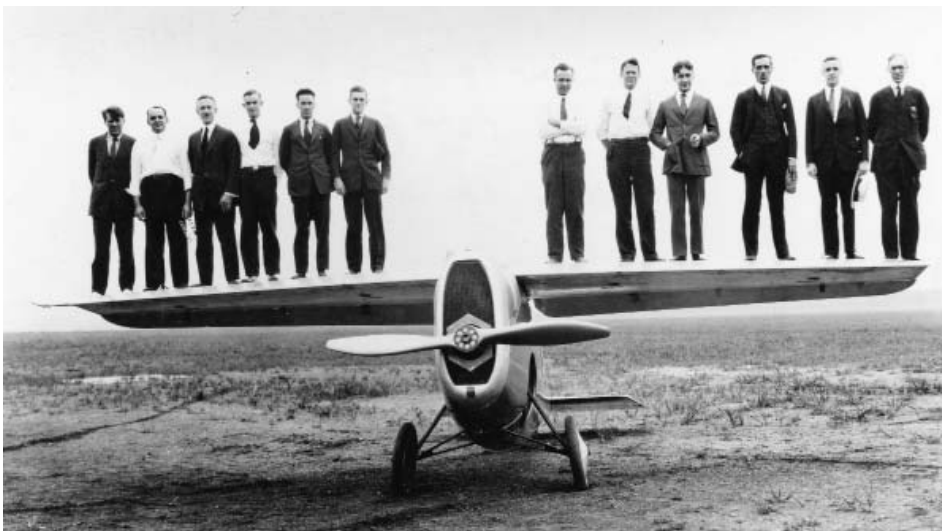
Another photo of the RB-1 undergoing a negative 12-G (guys) stress test. The men standing on the wings are listed from right to left: Howard M. Rhinehart, James M. Jacobs, J. P. Henry, Harvey D. Geyer, Bernard L. Whelan, Wallace S. Whittaker, Thomas Midgley Jr., J. H. Hunt, Milton Clement Baumann (chief designer), Harold E. Talbott, G. M. Williams, and Charles F. Kettering. The RB-1 was also known as the Dayton-Wright Racer. (Photo courtesy of Special Collections and Archives, Wright State University, MS152-217)
