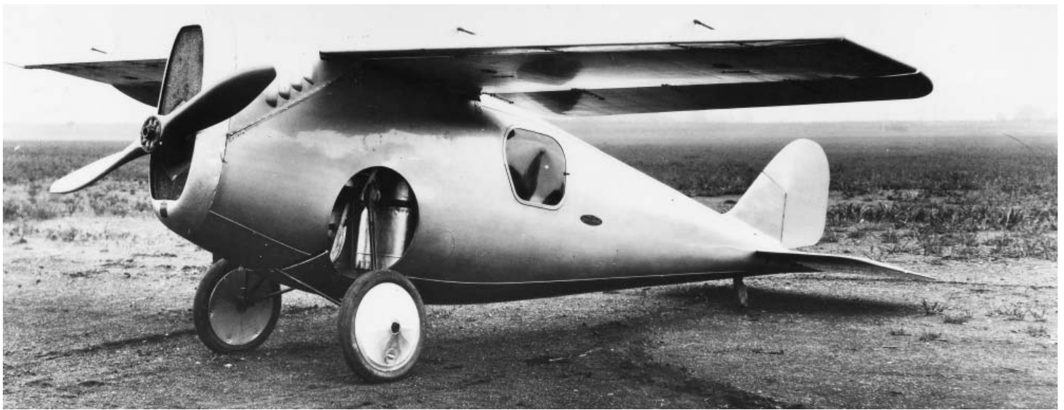
The RB-1 was revolutionary in design featuring retractable landing gear, a fully cantilevered solid-core variable-camber wing and full monocoque enclosed fuselage - features that would not regularly be incorporated in designs for another 10 years. Though it failed in the only race it was entered in, the plane still “caught the eyes” of many in the industry. It survives today on display at the Henry Ford Museum in Dearborn, Michigan. (Photo courtesy of Special Collections and Archives, Wright State University, MS152-207)
