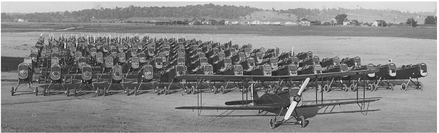
Approximately 150 completed DH-4 fuselages arranged on South Field. At the height of production, this represents about five days of production by Dayton-Wright. (Photo courtesy of Special Collections and Archives, Wright State University, MS152-53)
