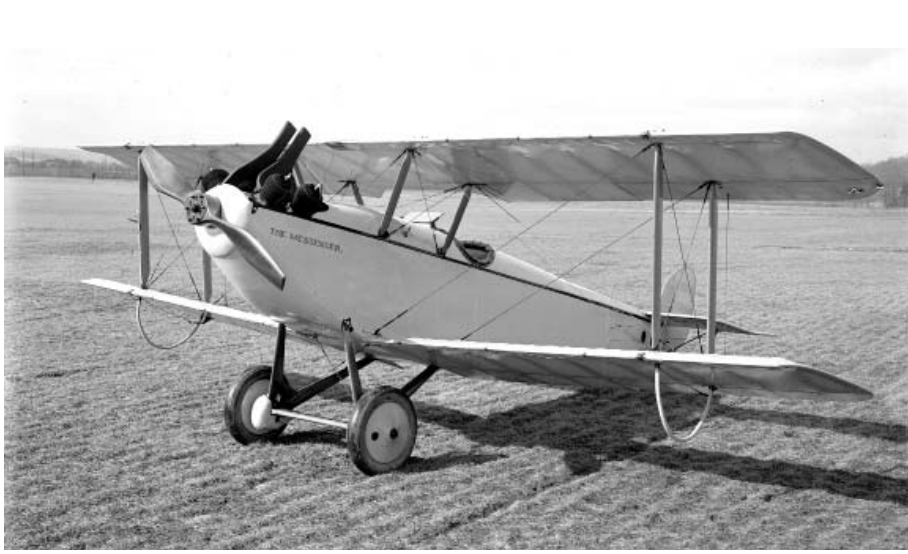
The Dayton-Wright T-4 Messenger was developed as an engine-test platform, though it was given a cover story that persists to this day. (Photo courtesy of Special Collections and Archives, Wright State University, MS152-131)
