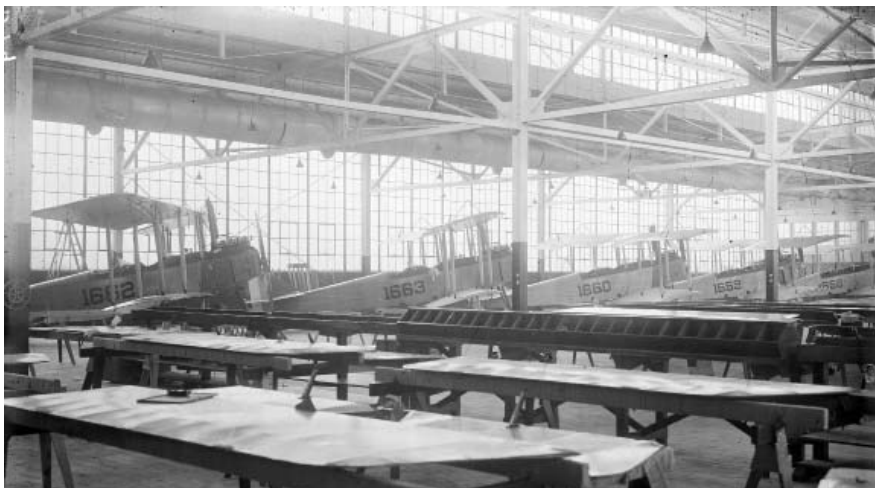
The Standard J-1 production line at Dayton-Wright's Plant 1 in Moraine, Ohio. (Photo courtesy of Special Collections and Archives, Wright State University, MS152-193)
