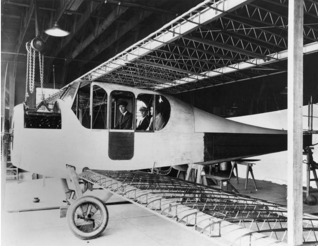
The OW-1 Aerial Coupe was the last aircraft designed by Orville Wright. Featuring an enclosed cabin, this four-place design set an altitude record of 19,710 feet on May 22, 1921, with D-W test pilot Bernard L. Whelan at the controls and three passengers on board. Seen here during construction with Bernard Whelan sitting in the pilot's seat and two unidentified people in the passenger seats. (Photo courtesy of Special Collections and Archives, Wright State University, MS152-208)
