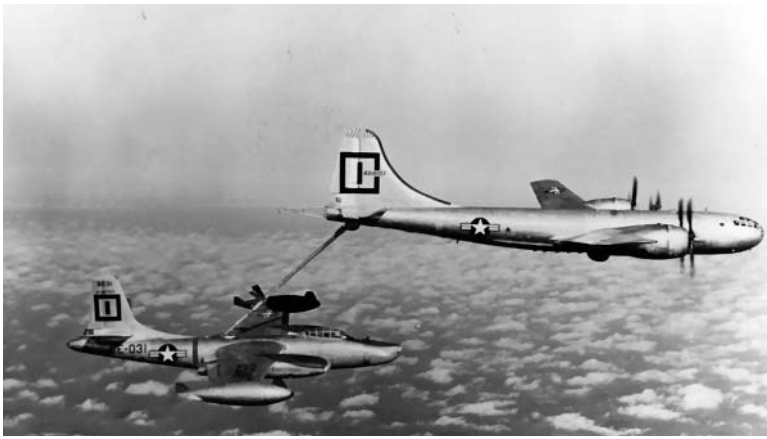
A 91st Air Refueling Sqdn. KB-29P from Barksdale AFB, La., refuels an RB-45C of the 91st Strategic Reconnaissance Wing using the flying boom. (USAF)
