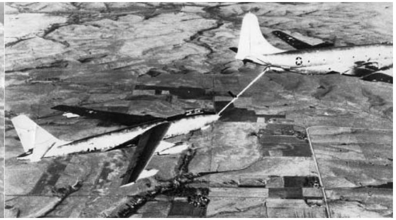
KC-97 tankers refueled Strategic Air Command B-47 force through the 1950s, using the flying boom. (USAF)
