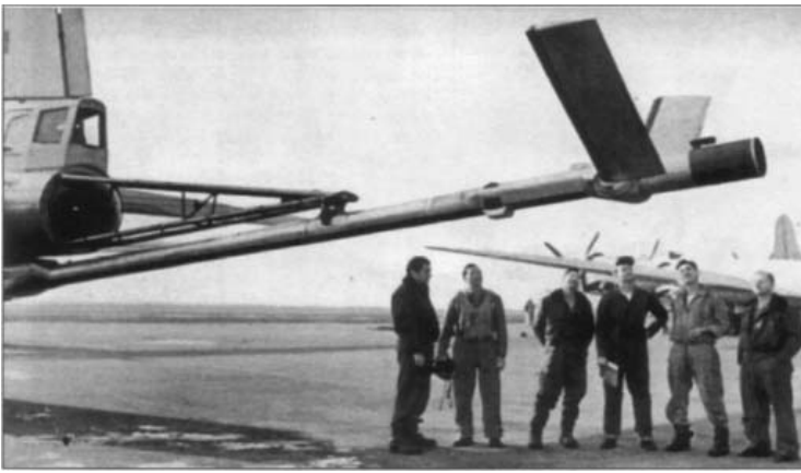
The "Boeing boom" offered greater fuel flow rates than the probe and drogue system and became the standard system for Strategic Air Command. (USAF)
