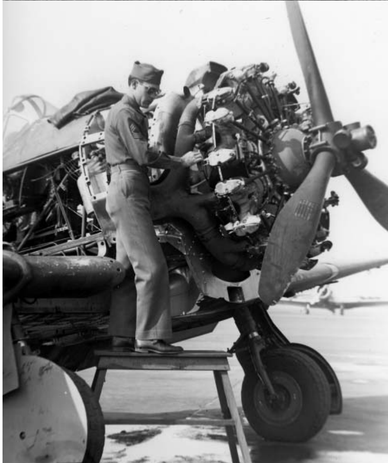
BOTTOM LEFT: Although this looks like a North American AT-6, it is not one! It is actually a North American P-64. It was one of six built for the Thai Air Force, but taken over by the U.S. Army Air Corps. Next to the sergeant's face is a tube where the machine gun barrel went. It was 1941 when this P-64 visited Parks Air College.
