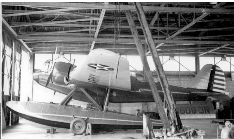
Martin YB-12A was adapted to floats to test its feasibility for use in coastal defense work.
