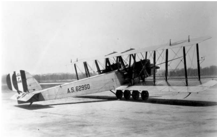
The WWI Martin MB-1 was the first bomber designed in the U.S. Its primary mission was as a reconnaissance scout plane for supporting ground forces with a secondary mission as a bomber.
