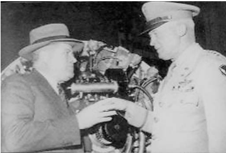
Chrysler was to begin engine delivery in March 1943 but there were start-up difficulties in buying the land, contracting the architects, and then construction that did start until June 1942. Chrysler then had problems obtaining engine blueprints and other data from Wright and crucial metals such as aluminum, steel and magnesium were in high demand and short supply. Chrysler President K.T. Keller (shown with Gen. Henry Arnold) was forced to ask for a July 1943 delivery date extension. (Chrysler)
