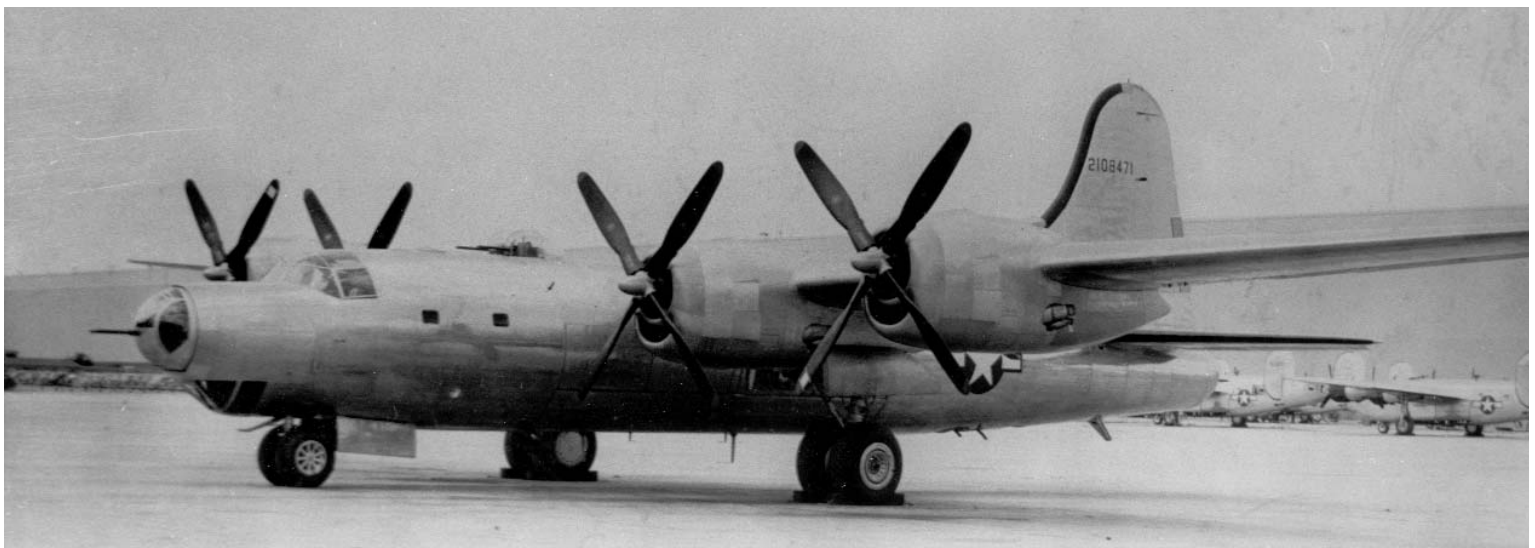
Consolidated XB-32-CF, 42-108471. The B-32 Dominator was ordered as a backup in case the B-29 program ran into insurmountable problems. The bomber also was powered by the R-3350 but ran into far fewer engine problems as the B-29 program, which had a higher priority status in development and testing, and the delayed B-32 program benefited from the previous B-29 engine problem solving. The B-32, however, suffered delays due to significant problems resulting from its initial tail design. (USAF photo from the Ed Stoltz collection, AAHS # P000144)
