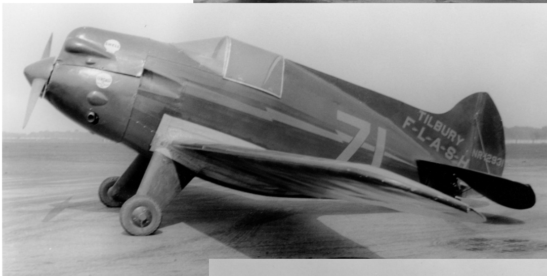
The Tilbury-Fundy "Flash," NR12931, race no. 71, competed in the small engine races at the 1934 National Air Races. The ship was flown by Clarence McArthur and was powered by a 4-cylinder, 45-hp Church 200 cu. in. engine.
