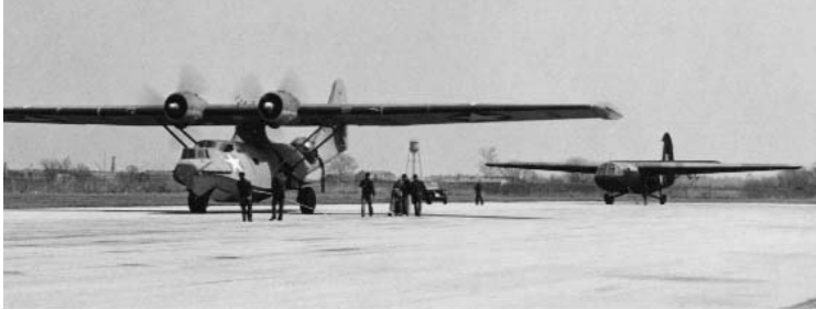
Another extraordinary image is this showing the NAF's Catalina standing by to take up tow line slack and pull a British Horsa assault glider into the air. One thing the tow tests of these large gliders made clear is that early notions of pulling three amphibious transport gliders behind twin-engine airplanes was fanciful. (National Soaring Museum)
