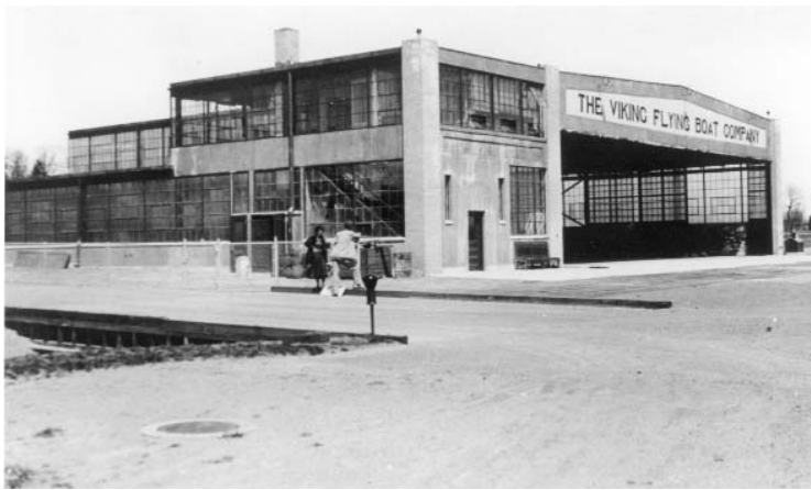
The Viking Flying Boat Hangar, circa 1938, New Haven Municipal Airport. (Photo from the Ev Cassagneres collection)
