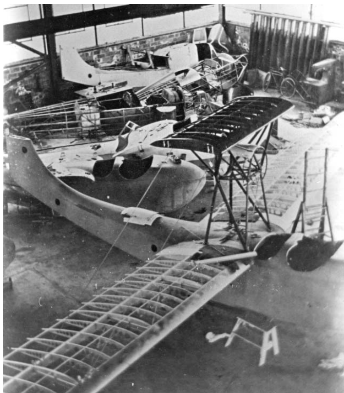
Viking flying boat under construction for USCG, in the hangar at New Haven Airport. Notice flying boat hull (cabin type) in corner. It was brought over from France before building up the Viking ships and never flew. It was lost in an explosion at Morris Cove, while starting its engine. (Photo from the Watson Bentley collection)
