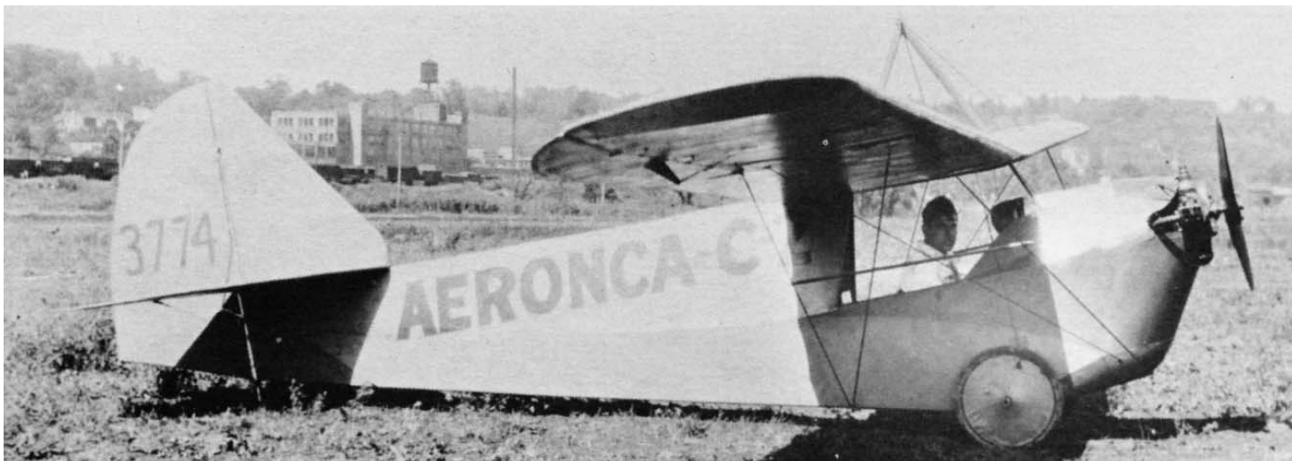
Rare photo of first Aeronca (more or less): the Roché-Dohse Flying Flivver, shortly after modification to the Aeronca C-2 form intended for mass-production. Incredibly, it was flown to over 20,000 feet by a test pilot, yet was first flown by someone who'd never flown a plane before. This tiny landmark plane now hangs in the Smithsonian's National Air & Space Museum, in the huge new Udvar-Hazy Annex, at Dulles Airport, Washington, D.C. -- a testament to its giant role in shaping personal aviation. (From Aeronca: A Photo History , by Hollenbaugh & Houser)
